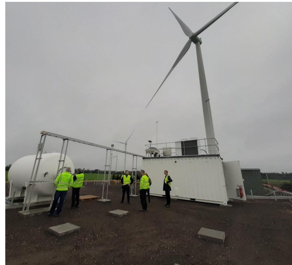
Electrolyzer and Buffer Tank (Week 38)
