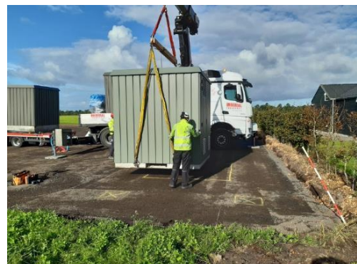
Transformer Station (week36)
