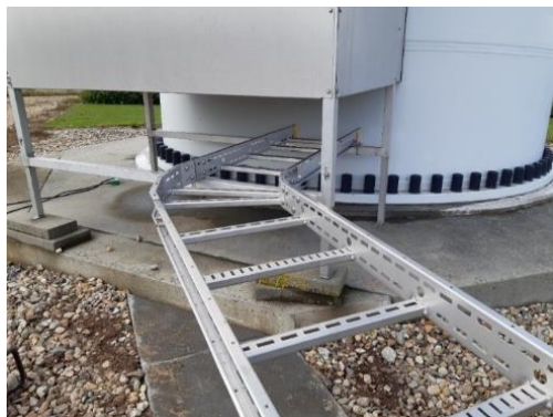
Cable Ladder (week35)
